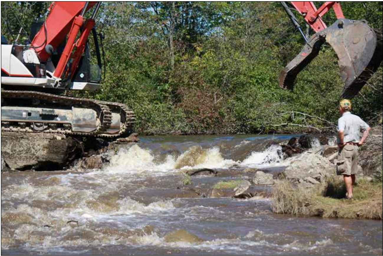
Removing a derelict dam reconnected the Kennebunk River with 7 miles of brook habitat for the first time in at least six decades.
